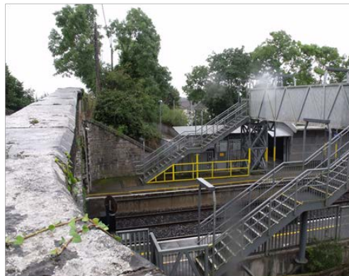
Confey Station to west of bridge
