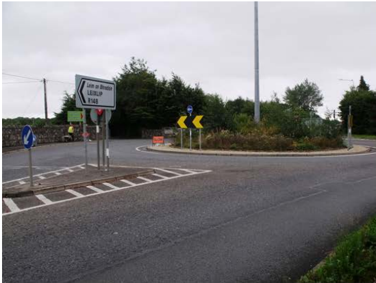
Roundabout on R148 at Junction 5
