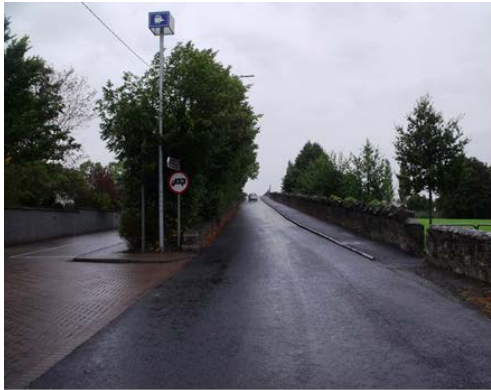
South side of Cope Bridge
