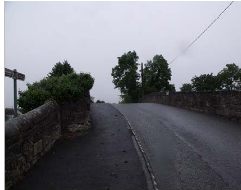
Crown of bridge
