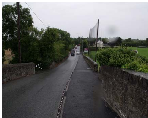
North side of Cope Bridge
