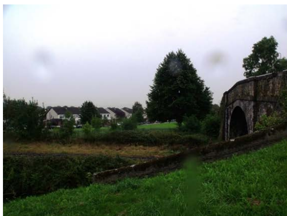
Eastern side of Cope Bridge, looking towards Glendale
