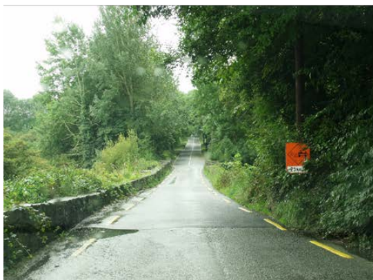
View of restricted Sandford's Bridge - with 1-way Yield
