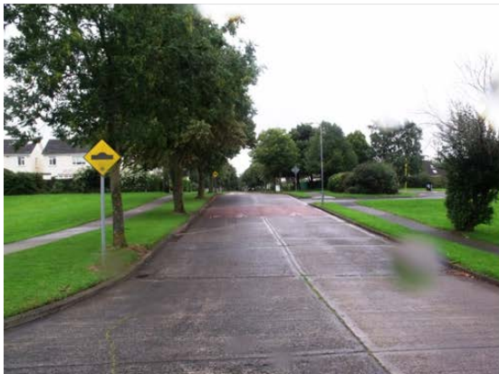
Main road through River Forest
